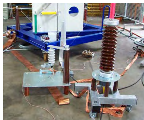
Impulse current testing arrangement for MV arresters
