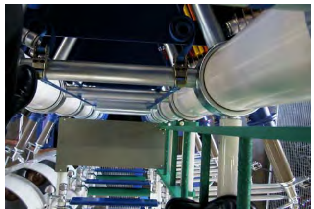
Internal view of ladder and platform
